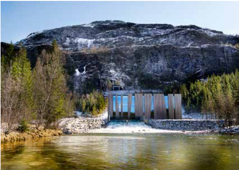
The Ovre Forsland power plant in Leirfjord, Norway. Credit: Innovation-Norway, Flickr, Licence CC BY-NC 2.0
