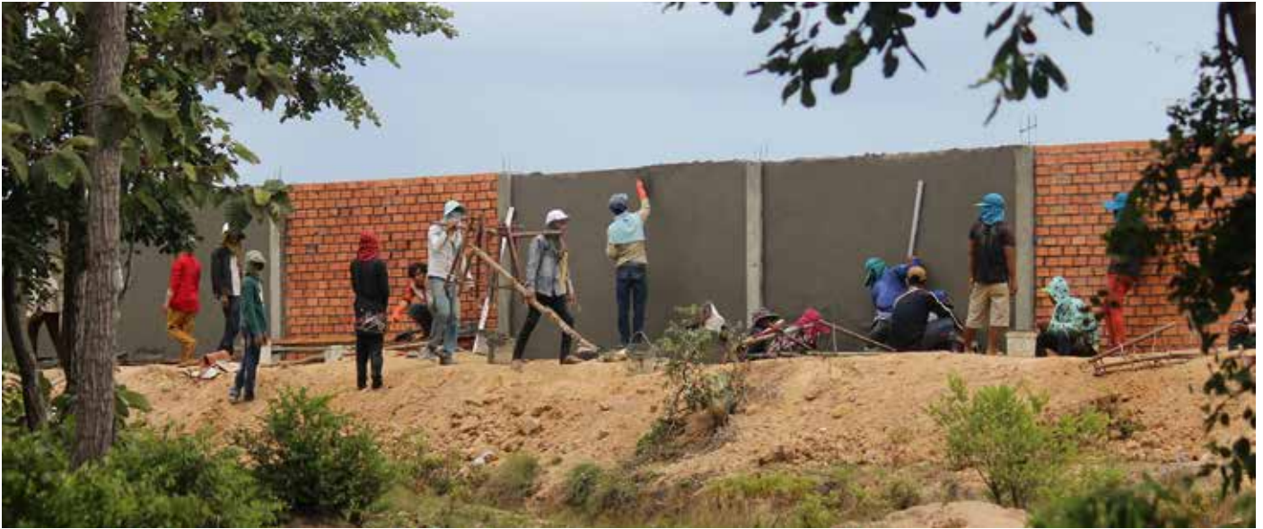
KDC company workers build the wall around the disputed land.
