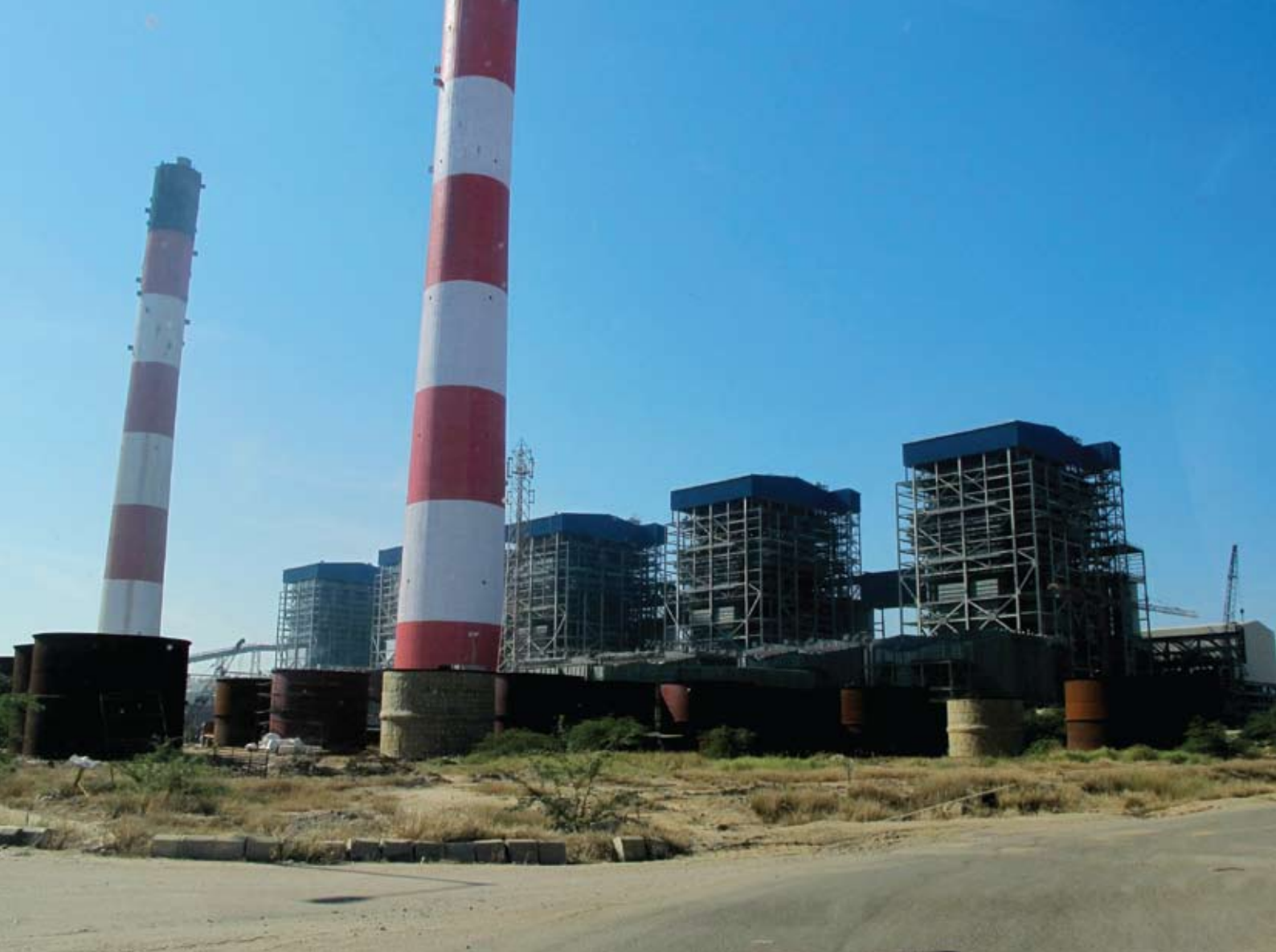
The under construction 4000 MW Tata CGPL Thermal plant in Mundra.
