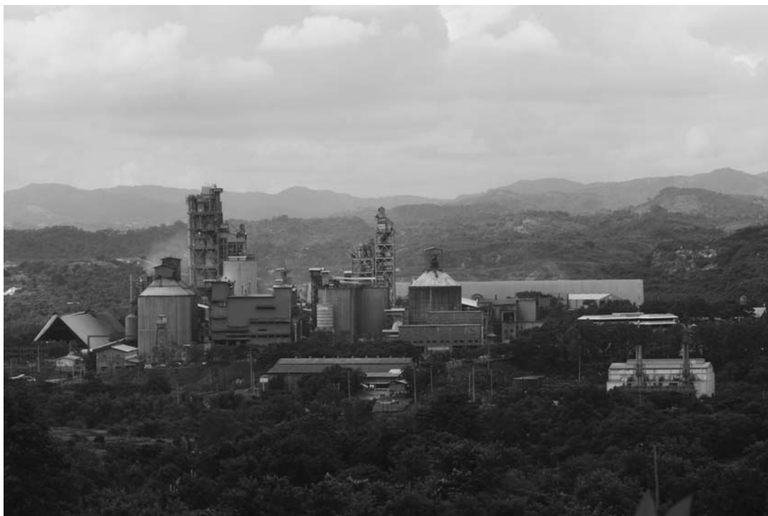
The Holcim cement plant in Bulacan hopes to earn additional revenues from the CDM by burning solid waste such as plastics and rubbers, in possible violation of the Clean Air Act ban on incineration. (By SONNY YABAO)
